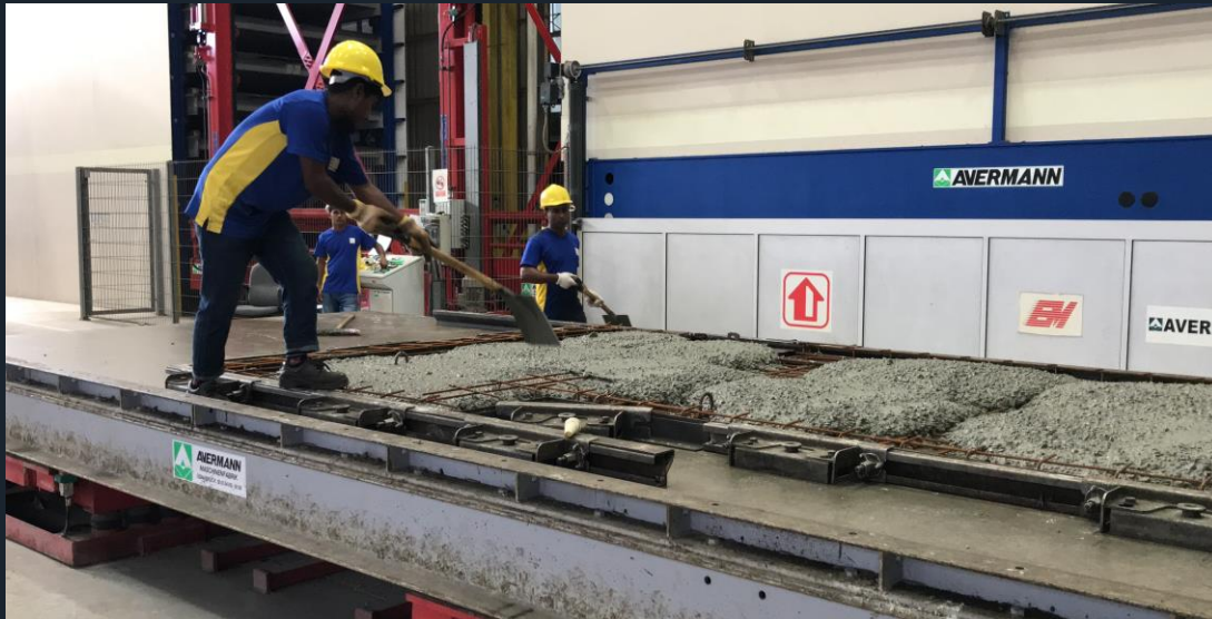
5. Spread wet concrete
